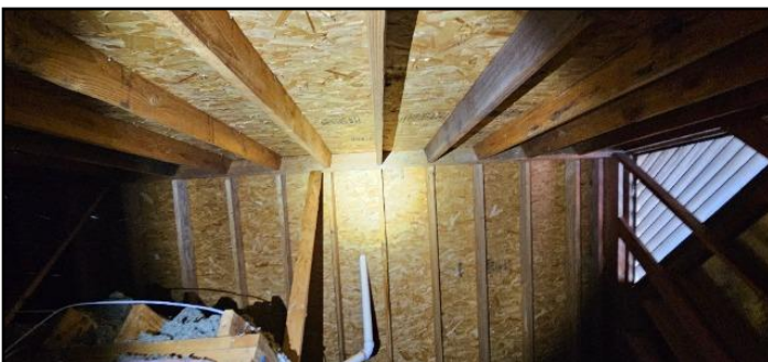
53. Rafters/ceiling joists
