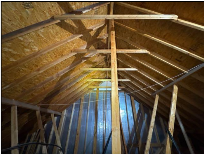
45. Rafters/ceiling joists
