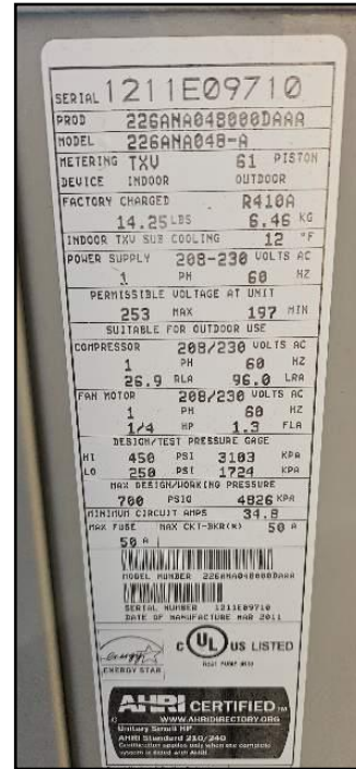
94. HVAC data plate
