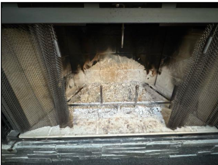
88. Inspect chimney, and sweep, if needed befor...
