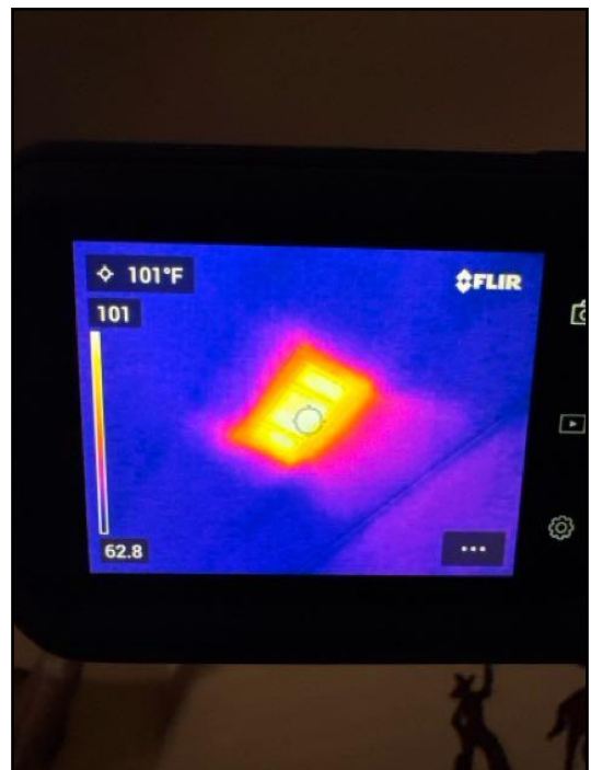
86. Heat pump operative
