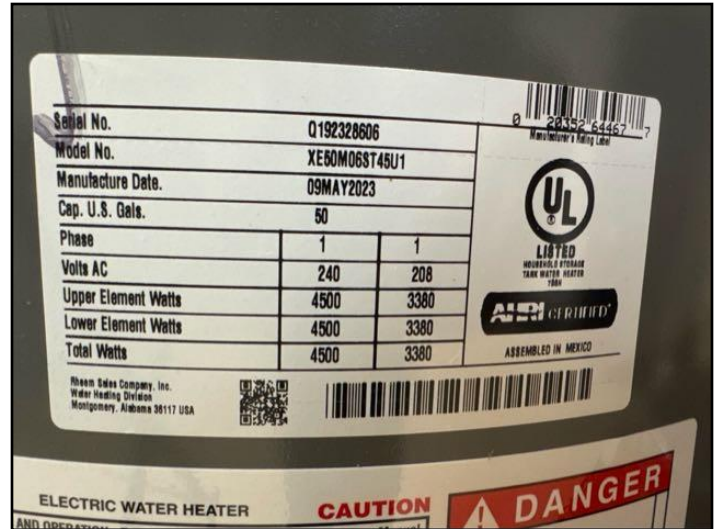
101. Water heater data plate
