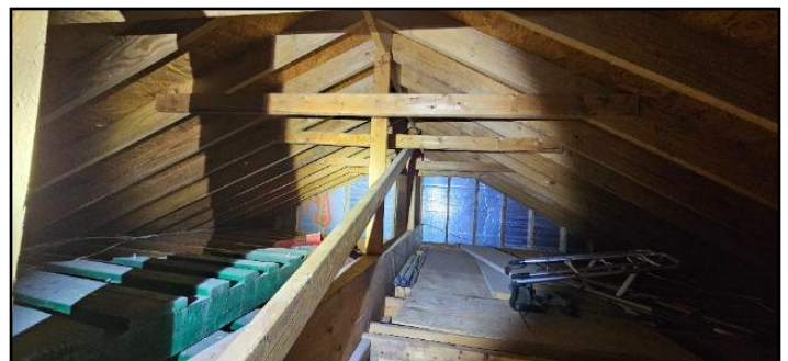
54. Rafters/ceiling joists
