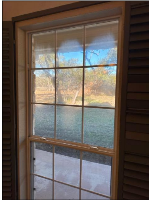
36. Lost seal on double or triple glazing
