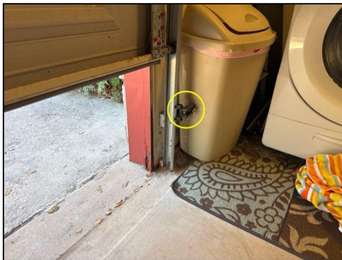
42. Photoelectric sensor more than 6 inches...
