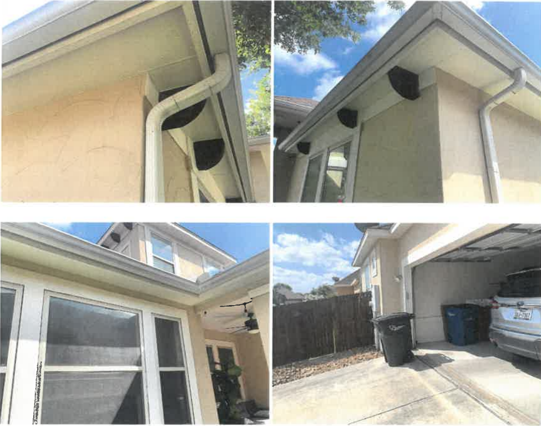
Pictures E3 - E6: General exterior pictures. No distress observed.
