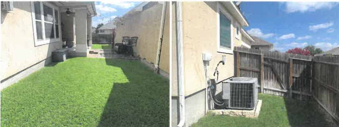
Pictures D3 and D4: Drainage along the right and rear.
