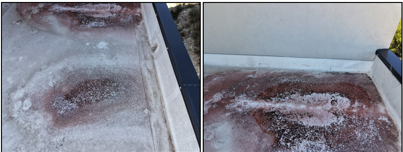
Signs of ponding observed at the flat roof covering.
