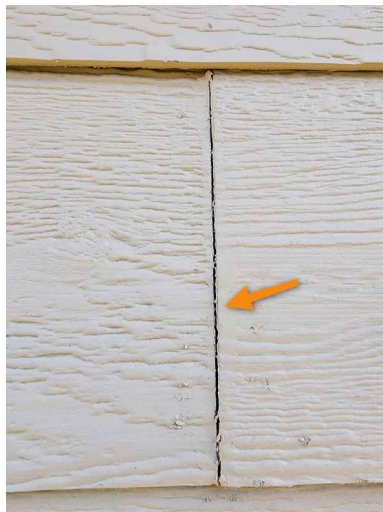
Throughout exterior wall
