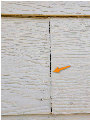
Throughout exterior wall
